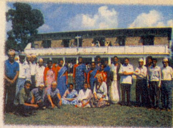
▲ THE LIBRARY Planning Committee stands in front of a school, as the library construction was underway.
